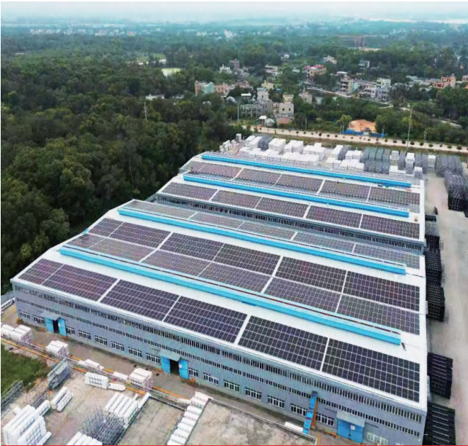
Dingan Roof Solar Power Station
