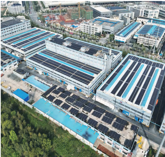
Changsha Roof Solar Power Station
