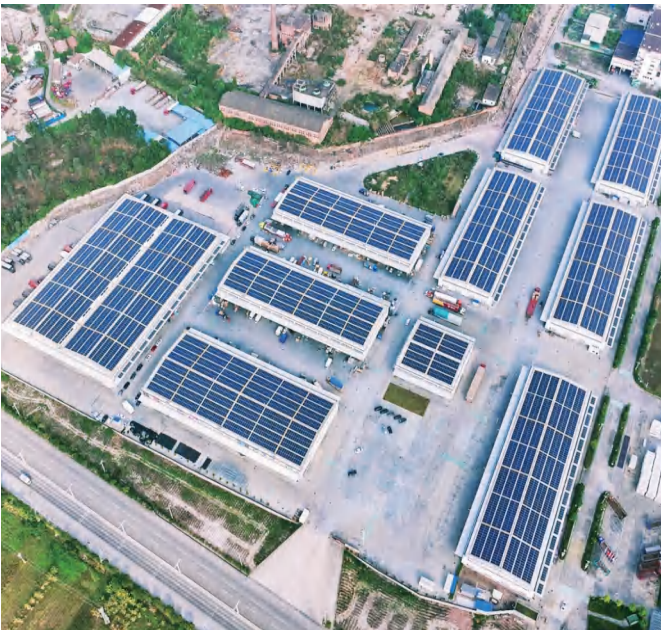
Maoming Logistics Roof Solar Power Station
