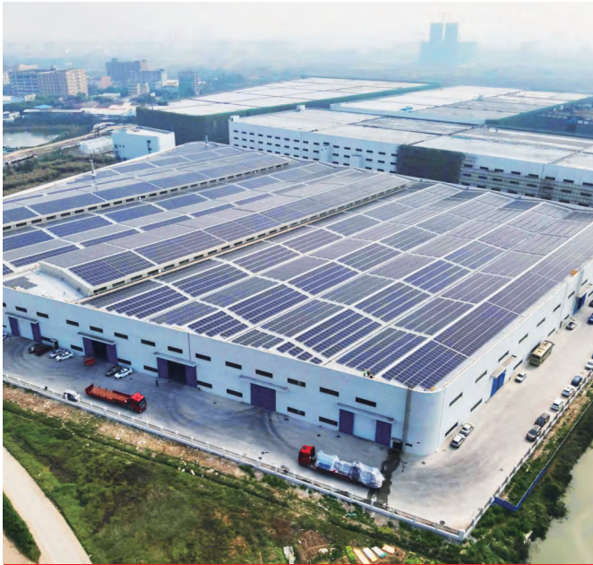
Haitian Roof Solar Power Station
