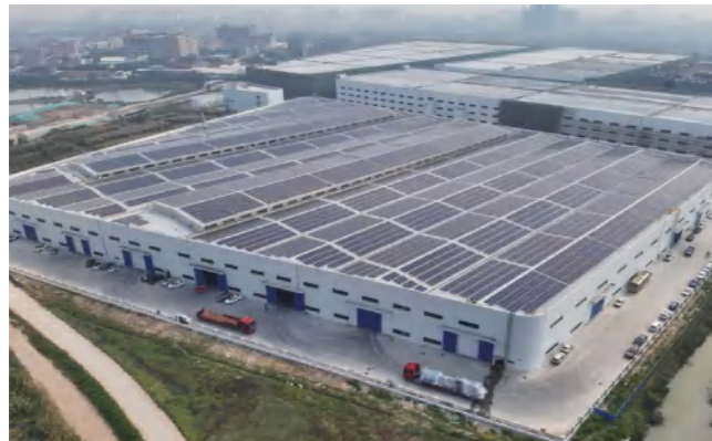
Foshan Haitian Roof Solar Power Station
