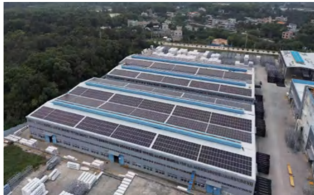
Dingan Roof Solar Power Station
