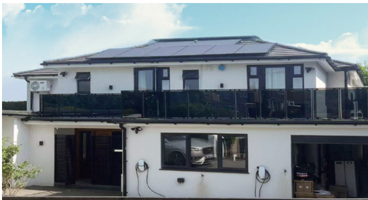
Location: Essex, UK | Project Capacity: 16.3kWp PV + 2x5kW Hybrid Inverters / 6x5kWh Batteries
