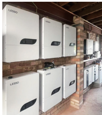
Location: Essex, UK | Project Capacity: 16.3kWp PV + 2x5kW Hybrid Inverters / 6x5kWh Batteries
