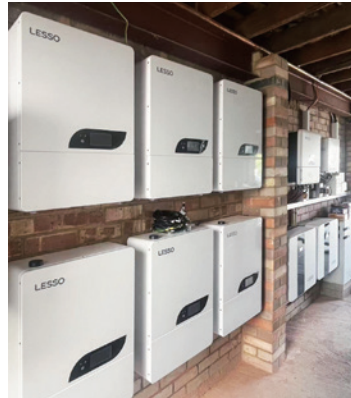
Location: Essex, UK | Project Capacity: 16.3kWp PV + 2x5kW Hybrid Inverters / 6x5kWh Batteries
