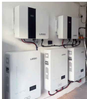
Location: Greater London, UK | Project Capacity: 2.2kWp PV + 2x5kW Hybrid Inverters / 3x10kWh Batteries
