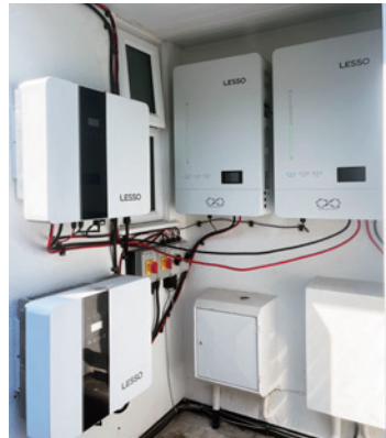
Location: Essex, UK | Project Capacity: 7.7kWp PV + 2x5kW Hybrid Inverters / 3x10kWh Batteries
