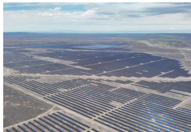
Karamay Desert Solar Power Station (Phase I)
