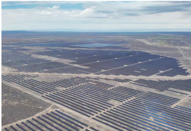
Karamay Desert Solar Power Station (Phase I)
