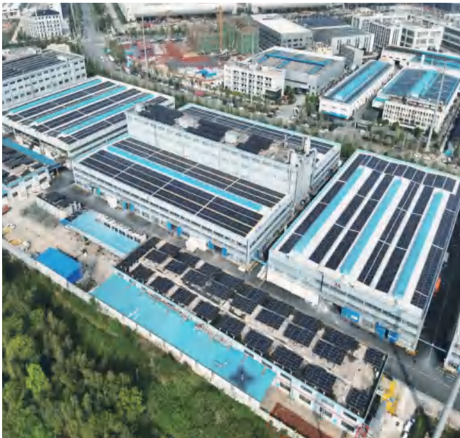
Changsha Roof Solar Power Station
