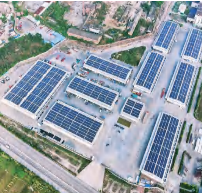
Maoming Logistics Roof Solar Power Station
