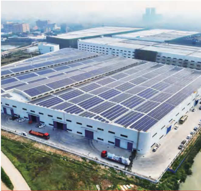
Haitian Roof Solar Power Station
